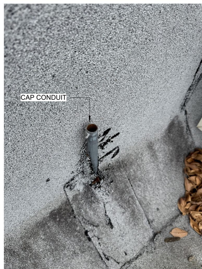
IMAGE THREE - OPEN CONDUIT
