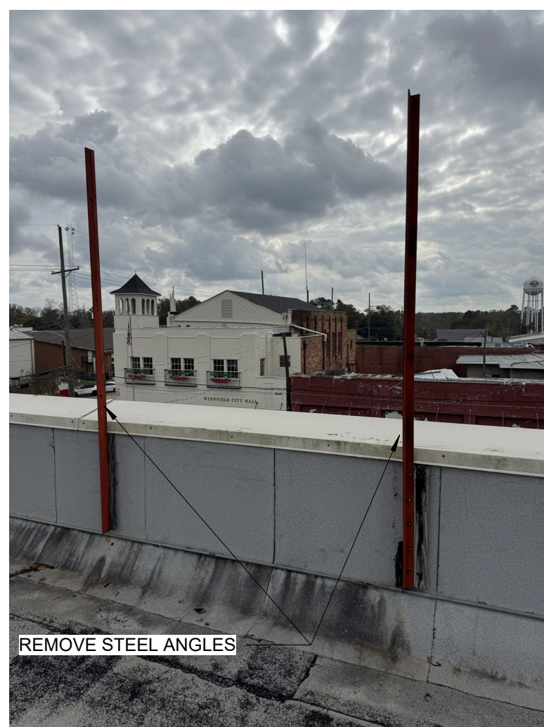
IMAGE FOUR - EXISTING STEEL ANGLES
