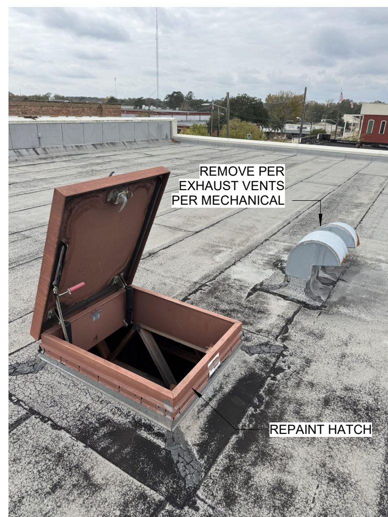
IMAGE SIX - EXISTING ROOF HATCH AND EXHAUST VENTS
