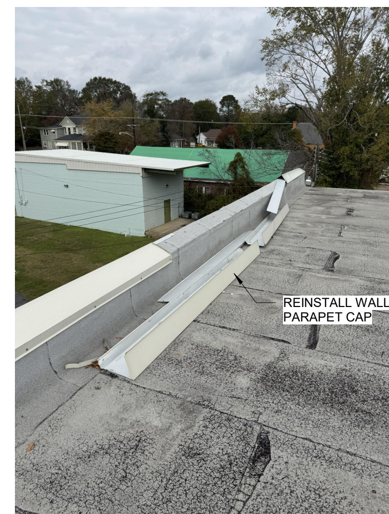
IMAGE SEVEN - EXISTING PARAPET COPING
