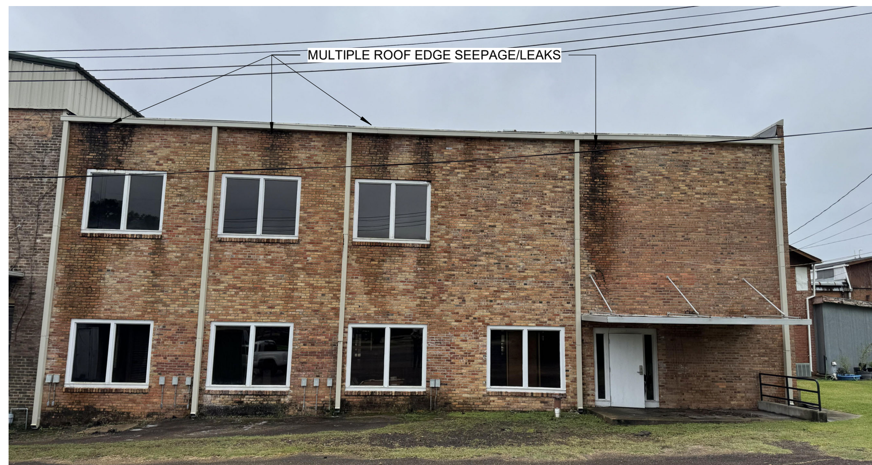
IMAGE ONE - REAR ELEVATION - ROOF EDGE/GUTTER LEAKAGE
