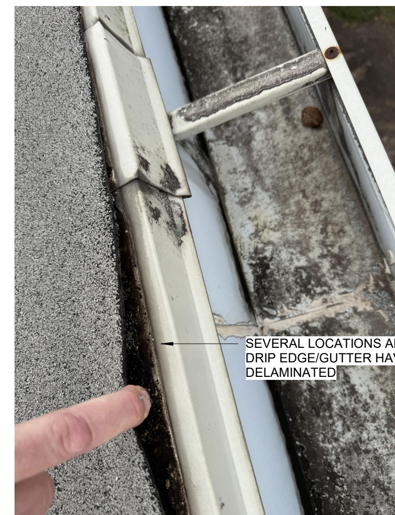
IMAGE TWO - ROOF DRIP EDGE/GUTTER
